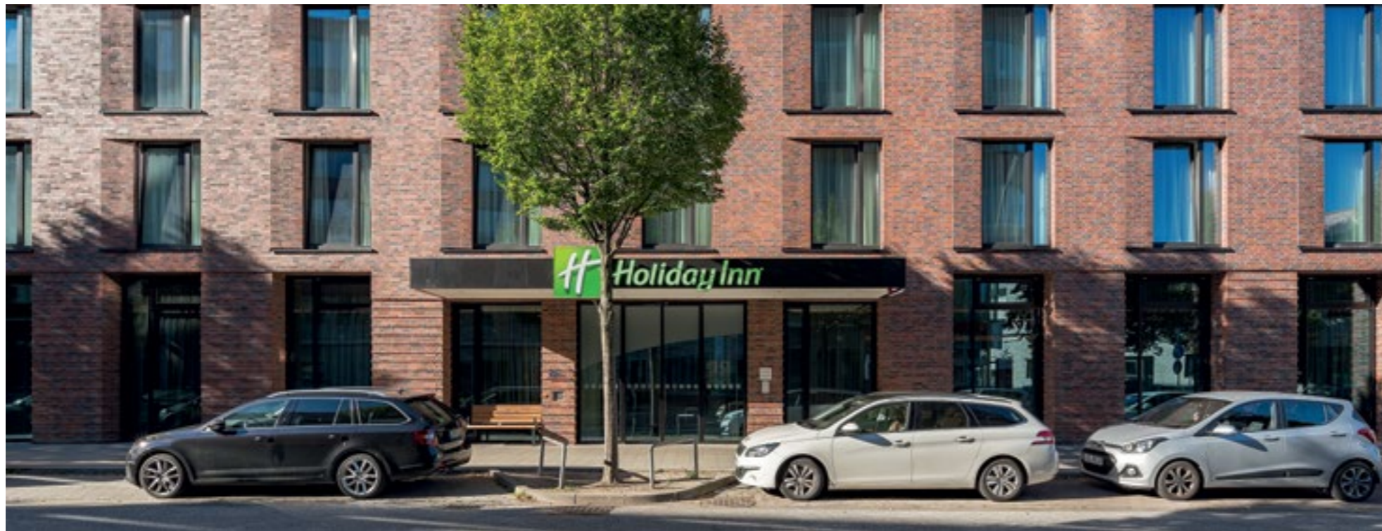
Holiday Inn Hotel, Hamburg, Germany. Project: www.mpp.de acquired by Vandersanden company
