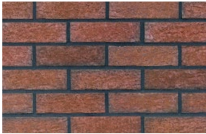
Tower bridge HF09
